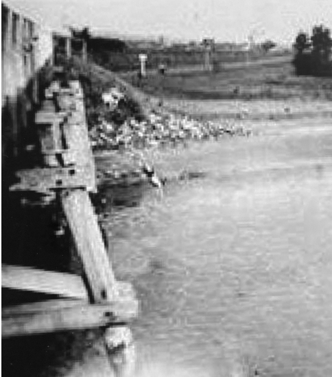
The first Canal bridge - all wooden structure.
