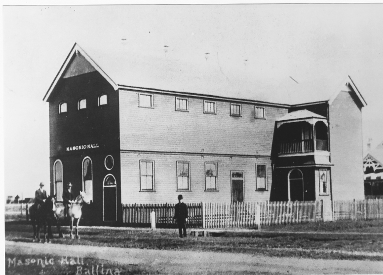
Masonic Hall before the balconies were added.
